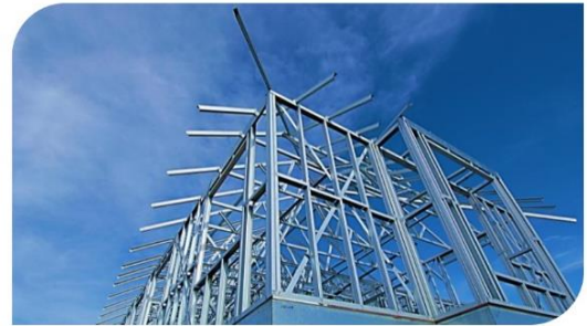
SMARTFRAME® light weight steel house framing application
