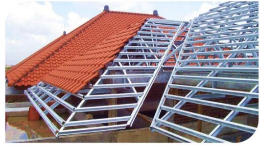
SMARTRUSS® light weight steel roof truss application
