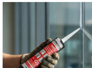
Instalasi Kaca Interior
