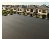
Dak Atap Beton
