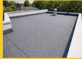
Dak Atap Beton
